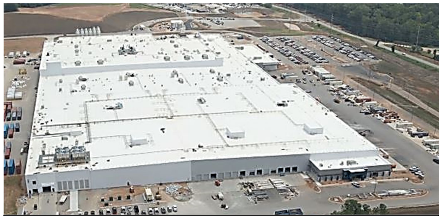
Aerial view of Smucker's plant under construction in July of 2023.
